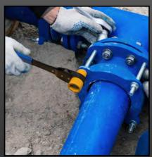
Wrenches are professional grade two in one tools for gas and water and most bonnet bolts.
