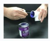
7. Using an aggressive scrubbing motion, apply the primer to the pipe end to just beyond the mark for the depth of the fitting socket.
