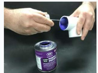
7. Using an aggressive scrubbing motion, apply the primer to the pipe end to just beyond the mark for the depth of the fitting socket.
