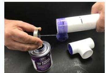
8. Apply second application of primer to fitting socket.
