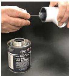
11. Apply a second coat of cement to the pipe end.
