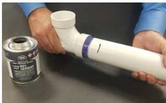
13. Hold pipe and fitting together to keep pipe from pushing out of fitting socket. Time will vary with pipe diameter, type of pvc cement, and ambient temperature.
