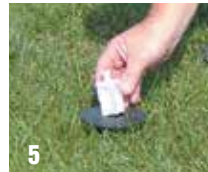
5 Insert lining peg into ground socket.
