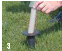
3 Insert socket setter into ground socket.
