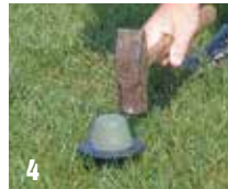
4 Using a rubber mallet or hammer, tap the socket setter until the ground socket is at the turf surface.
